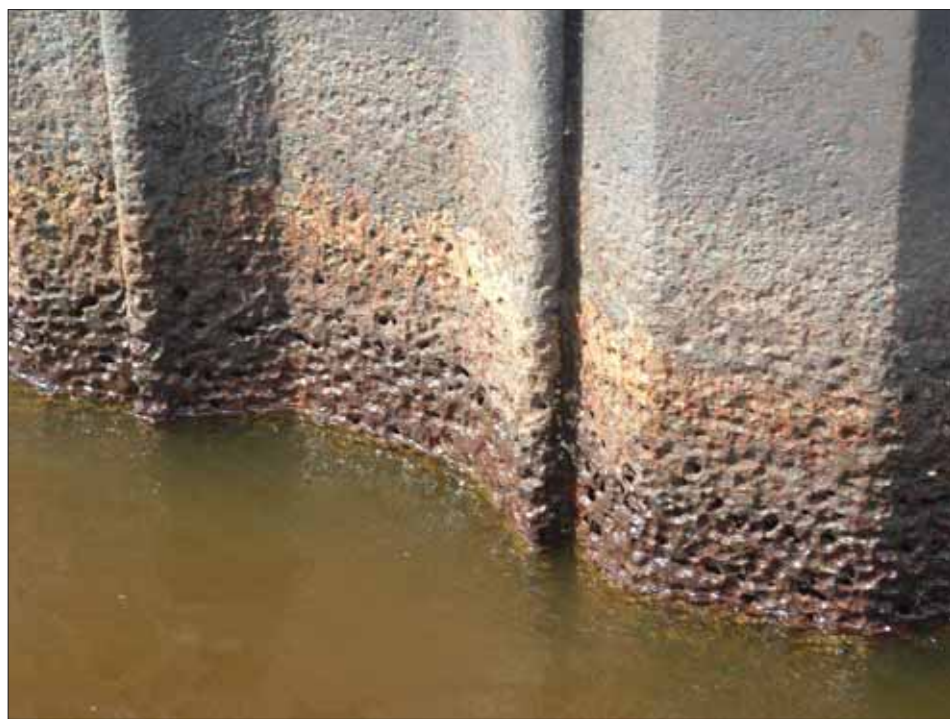
Corroding steel sheet-piling (and close-up) on the foundation of a navigation aid in the Duluth-Superior harbor, exposed during low water levels in 2007.
