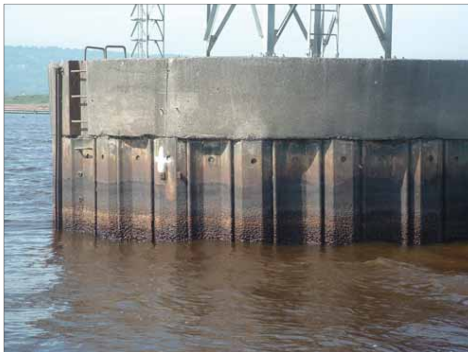
Corroding steel sheet-piling (and close-up) on the foundation of a navigation aid in the Duluth-Superior harbor, exposed during low water levels in 2007.
