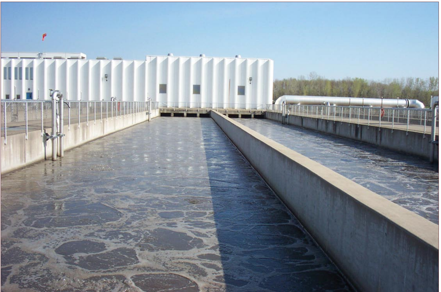
An aeration tank at a municipal wastewater treatment plant. The tank removes dissolved organic compounds by bubbling air through the wastewater, creating favorable conditions for the growth of bacteria that are capable of metabolizing pollutants.
